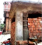
Figure 2. (a) Protest during Rani Pokhari Reconstruction (Source: The Kathmandu Post) and (b) Use of Concrete Post and Brick in Pati (Credit: Ar. Anil Tuladhar)
